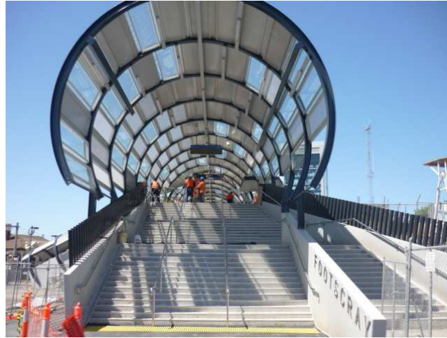
Main structure in location nearing completion.
