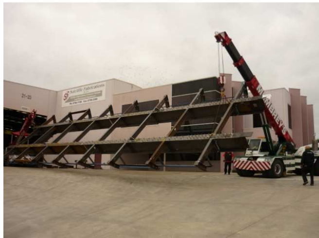
Craning the deck out of the factory for transport to site.
