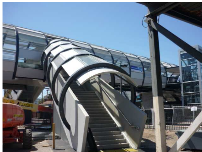
Side entries nearing completion.
