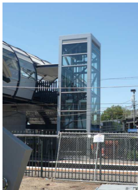
Completed lift at Footscray.
