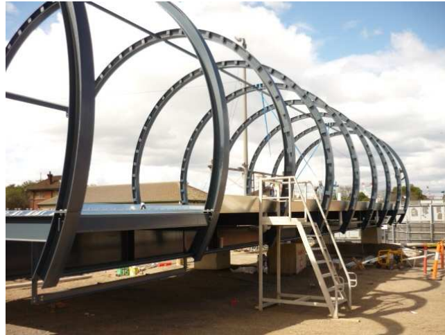
Assembly on site prior to lifting.
